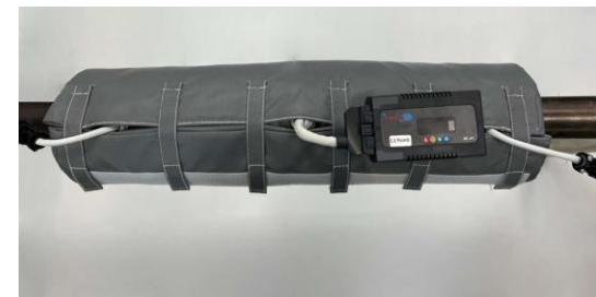
Heating jacket (Existing)
